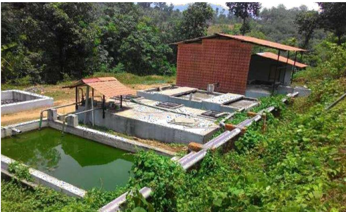
Figure 23: Sewage Treatment Plant – Overview
