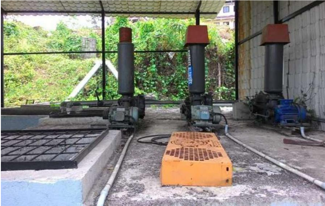
Figure 24: Sewage Treatment Plant- Motors
