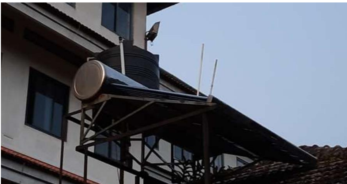
Figure 7: Solar Water Heater Units
