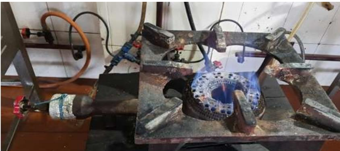
Figure 9: Bio Gas Stove and units
