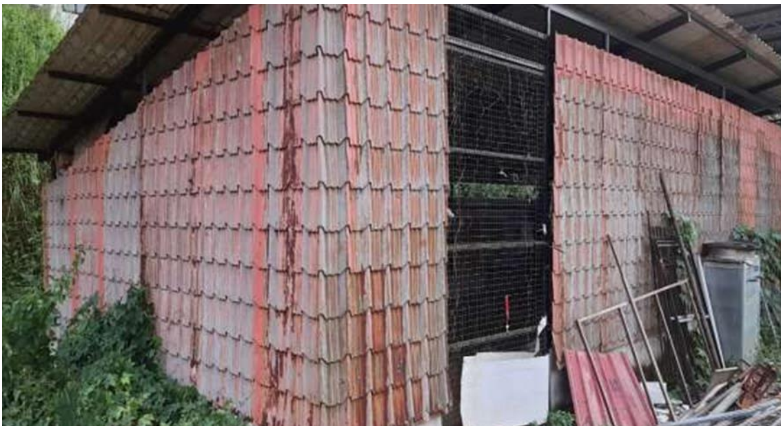
Figure 28: Solid Waste warehouse
