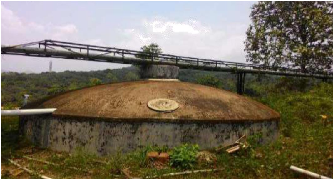
Figure 12: Rain Water Harvesting Tank- Alphonsa Hostel
