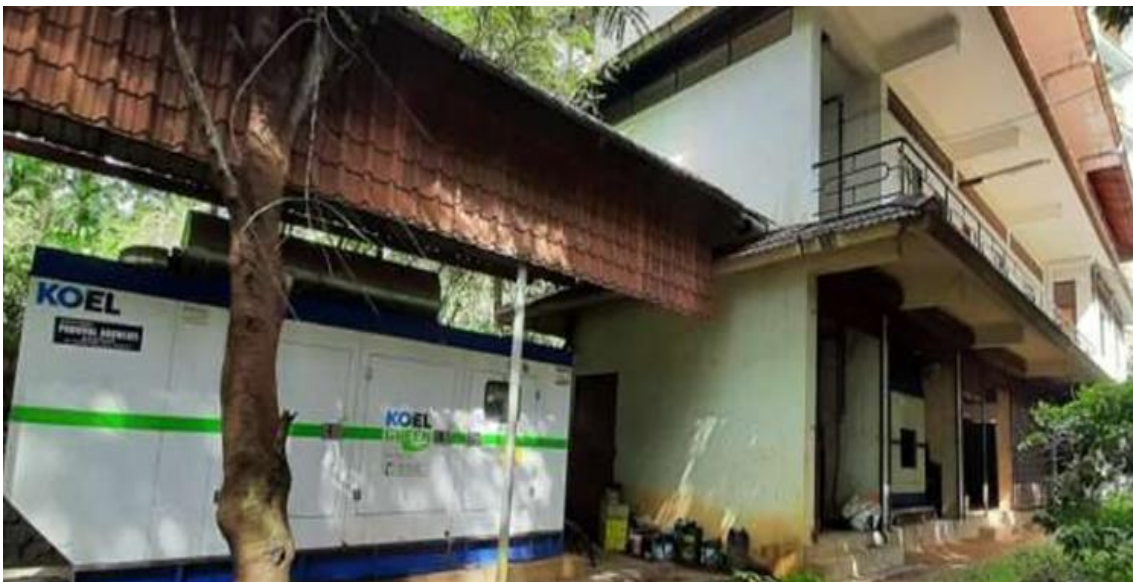
Figure 31: Eco friendly Generator set at the Power house
