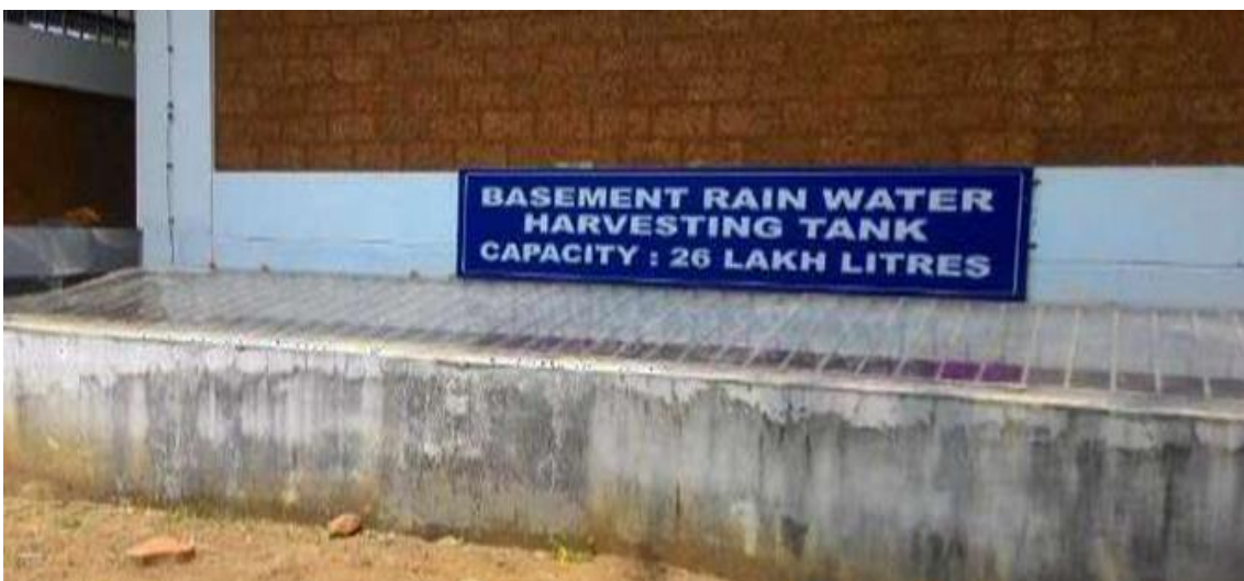
Figure 11: Rain Water Harvesting Basement Tank
