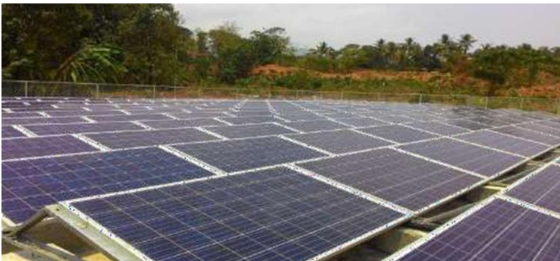
Figure 4: Solar Power Plant Panels near VJIM
