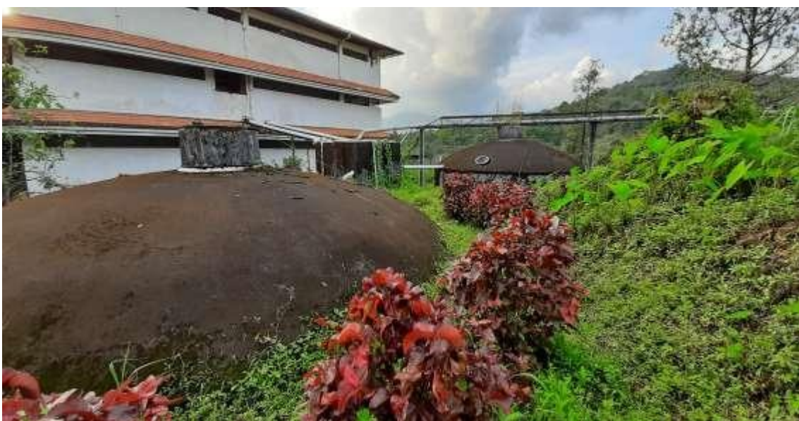
Figure 13: Rain Water Harvesting Tank- Near Sanjose and PG Hostels
