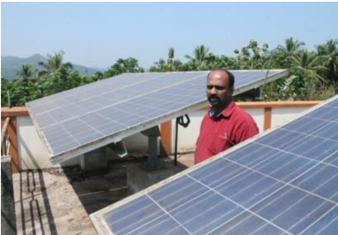
Figure 6: Solar Panel Unit- Rooftop project
