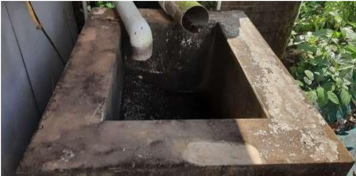
Figure 18: Rain Water well Recharge Filtering system
