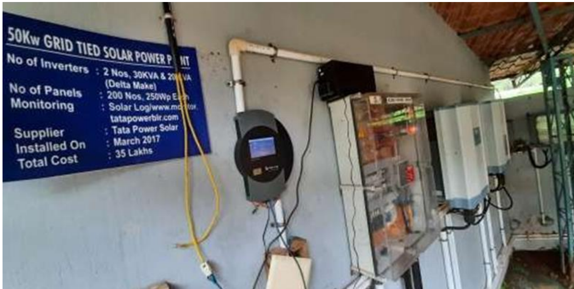
Figure 5: Solar Power Plant- on Grid control units
