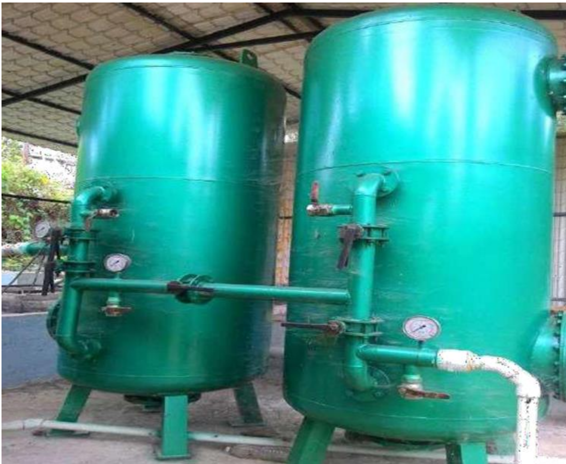
Figure 25: Sewage Treatment Plant- Filters
